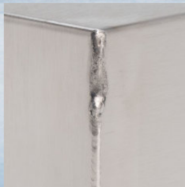
Manual welding with correction
